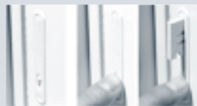
Operation of a vent latch
